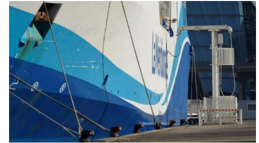
Electric connection – “Cold ironing”
